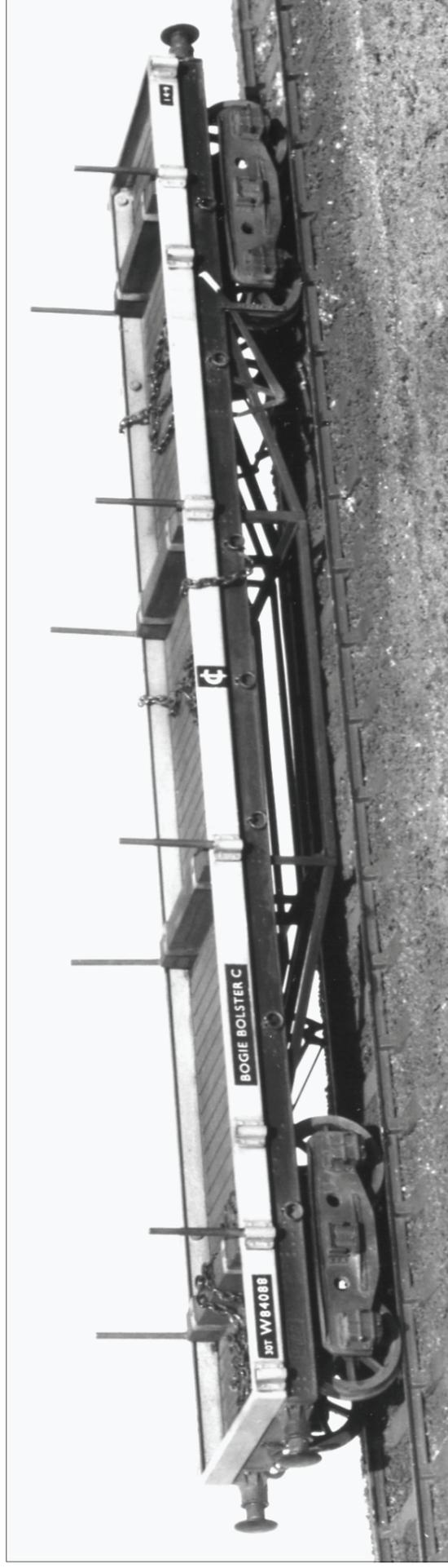
These heavyweight 30 ton 48 foot long bogie bolsters were built in considerable numbers from 1907 until early BR days. Originally intended as rail carrying vehicles for the P.W. department, but once the usefulness of the design became apparent they were used for all manner of loads.
